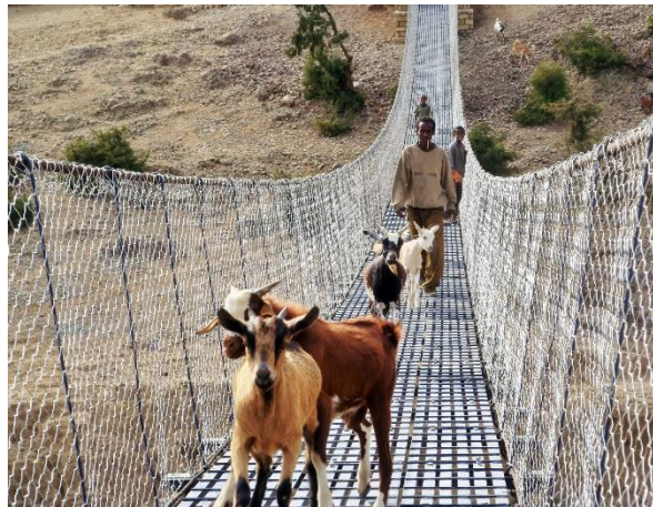
Adyem bridge, photo by Padam Gurung
