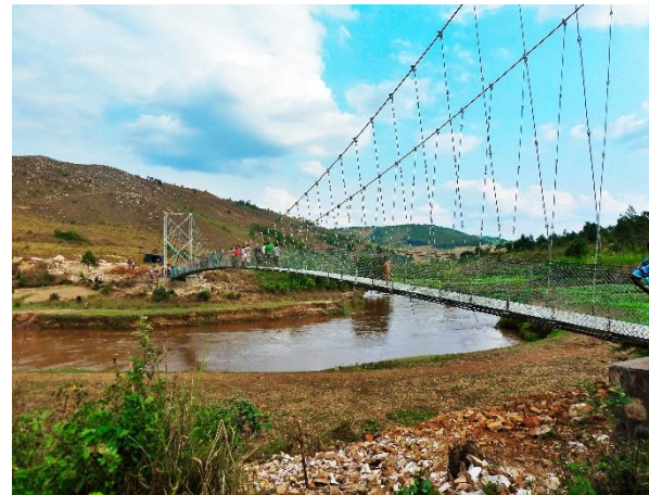
Ruvubu Bridge, photo by Padam Gurung
