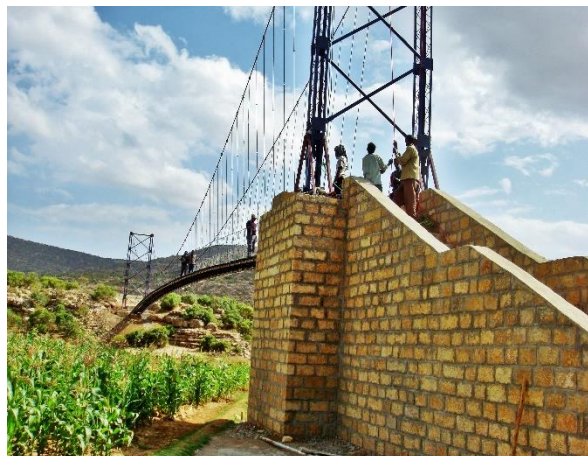
Endamino bridge, photo by Padam Gurung
