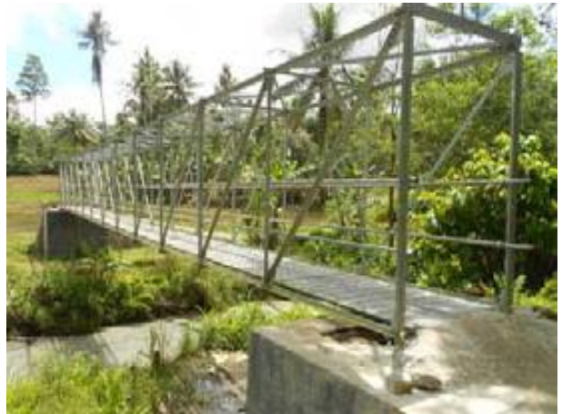
Baukhe Steel Truss Bridge, photo by Bindu Khumbu
