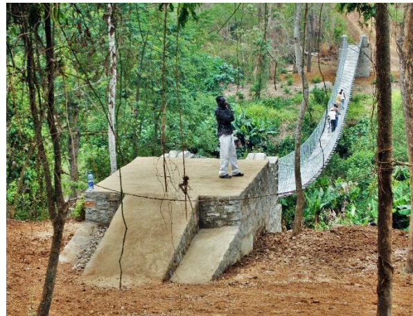
Srimajangar bridge, photo by Padam Gurung
